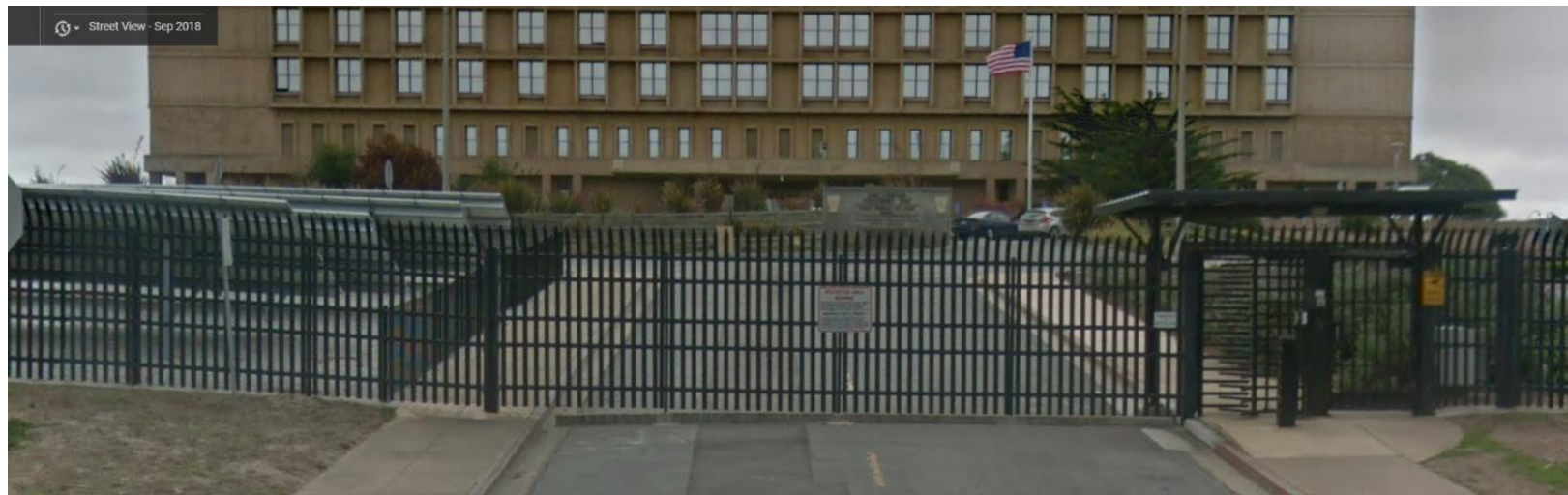
Photo 3: Example fence and gate at Department of Defense Center.
