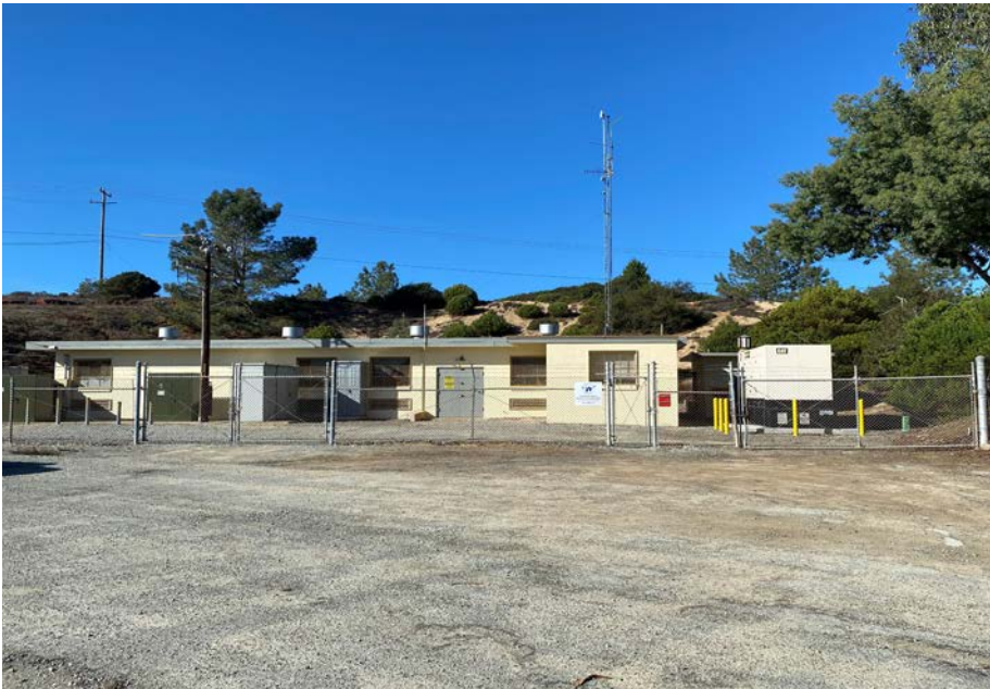
View of existing B/C BPS, looking west.
