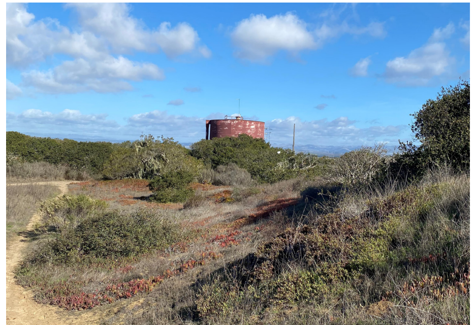
View of existing Intermediate Reservoir and surrounding vegetation, looking north.
